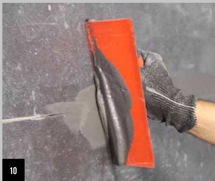
GROUTING AND FINAL CLEANING
